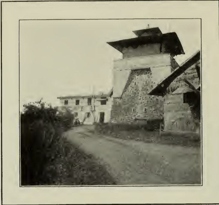
THE EXTERIOR OF TOWER TELEGRAPH OFFICE IN AN OLD FORT.
